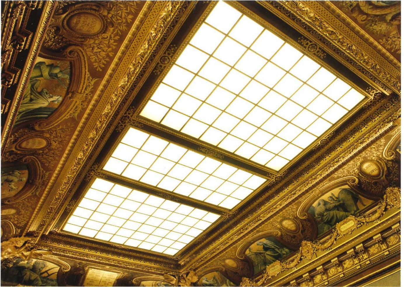
**Above:** Restoration of the glass roof (5 x 11 meters) lighting the General Assembly Room in the Conseil d'État, Paris. The steel framework was filled in with a brass grid and frosted glass.
